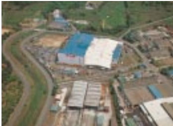
Denyo Shiga Plant, Japan
